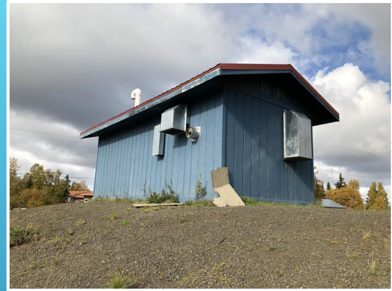
Nearly Complete Lift Station
