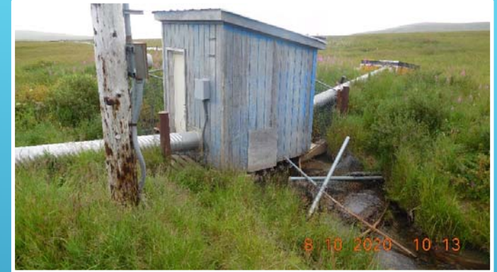
Unnamed Creek Intake
