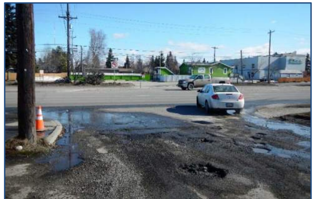
Intersection of Minnesota Drive and W. 32nd Avenue – deteriorating pavement and sight line issues.
