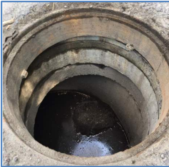
Photo 3 - Frame, Grade Rings & Reducing Slab
