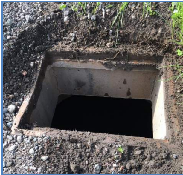
Photo 3 - Frame & Reducing Slab
