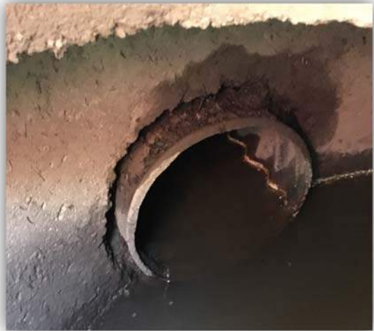
Photo 3 - Grout Loss at Pipe Penetration
