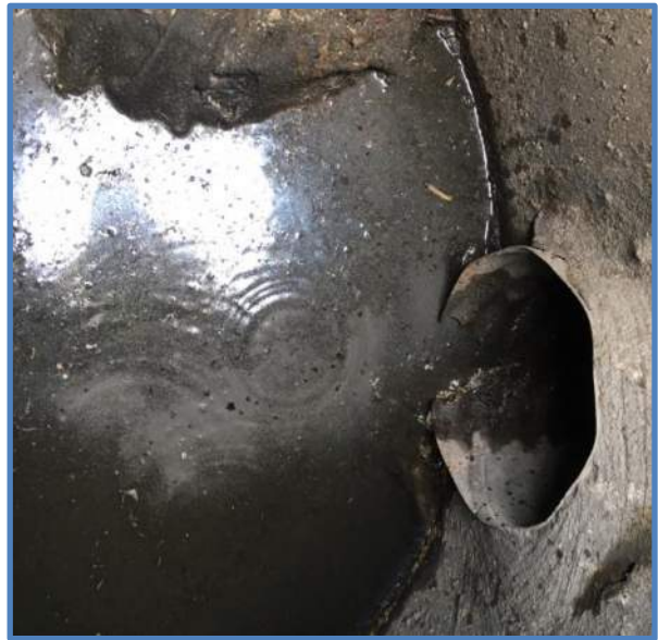
Photo 4 - Outlet Pipe Penetration
