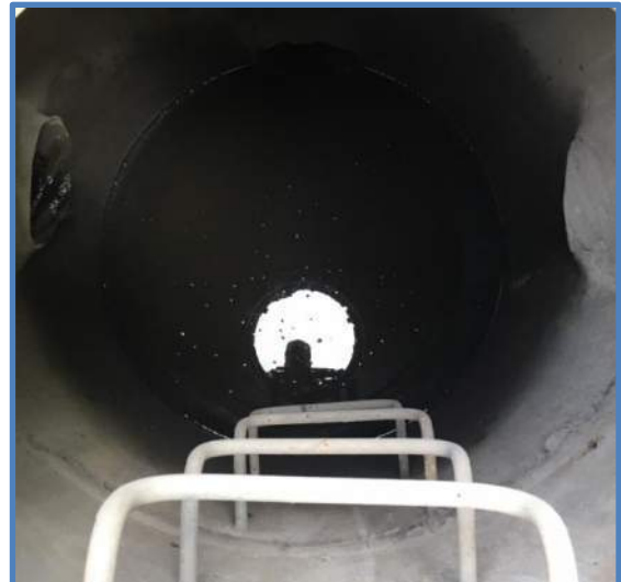
Photo 5 - Inlet & Outlet Pipe Penetrations & Ladder Rungs
