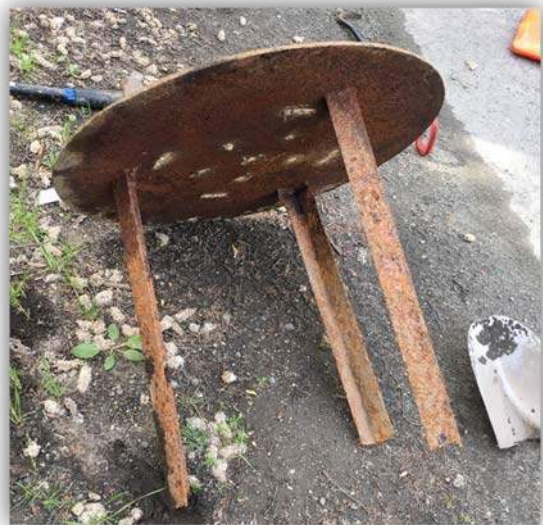
Photo 4 - Non-standard Manhole Lid
