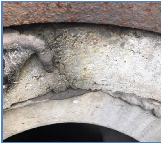
Photo 3 - Cracking in Grade Ring
