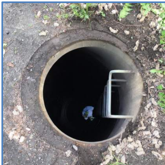
Photo 4 – Manhole Cone & Ladder Rungs
