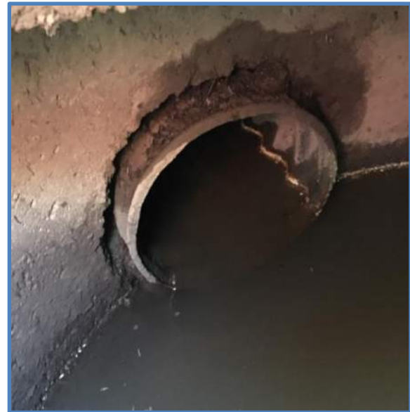
Photo 4 - Outlet Pipe Penetration
