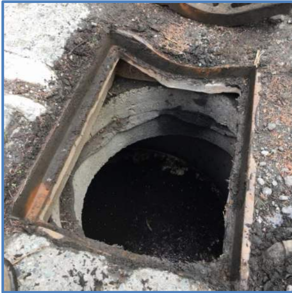
Photo 3 – Frame, Grade Rings & Reducing Slab
