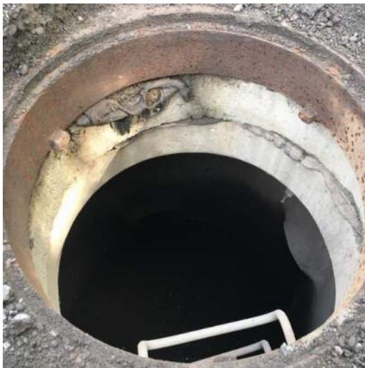
Photo 4 - Frame, Grade Ring & Manhole Cone
