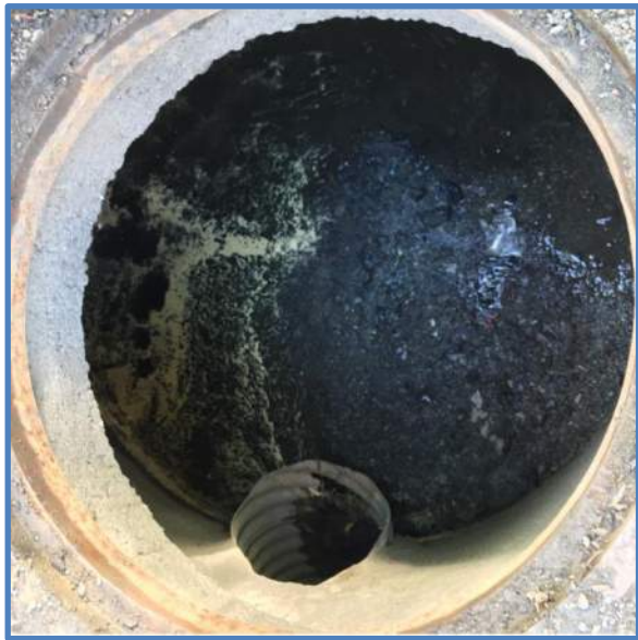
Photo 3 - Frame, Reducing Slab & Outlet Pipe
