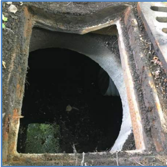
Photo 3 – Frame & Reducing Slab
