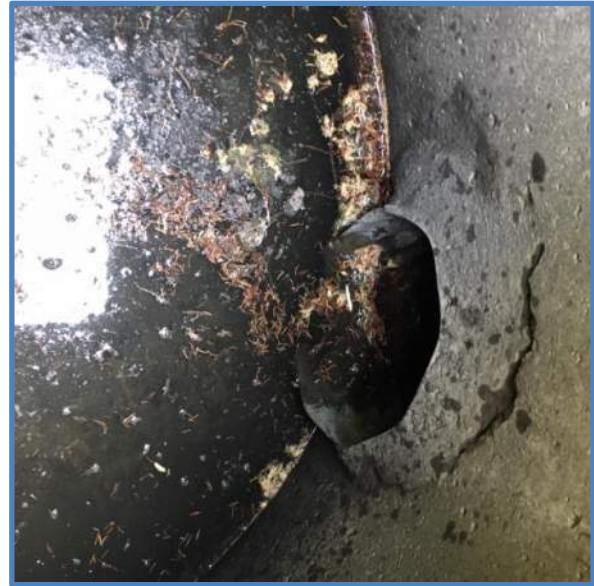
Photo 4 – Outlet Pipe Penetration
