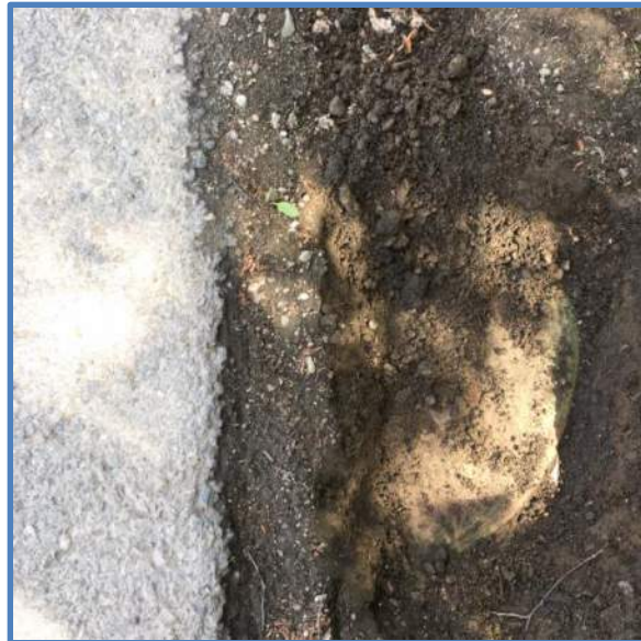
Photo 3 – Manhole Lid Under Pavement
