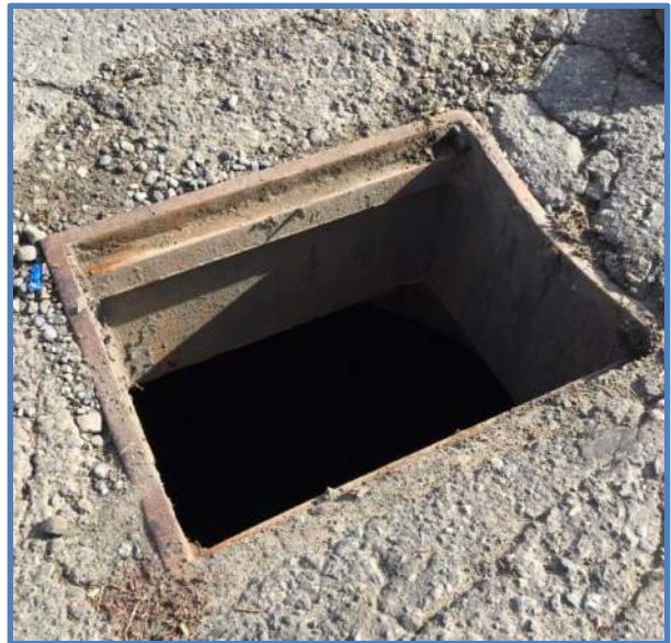
Photo 4 - Frame & Reducing Slab
