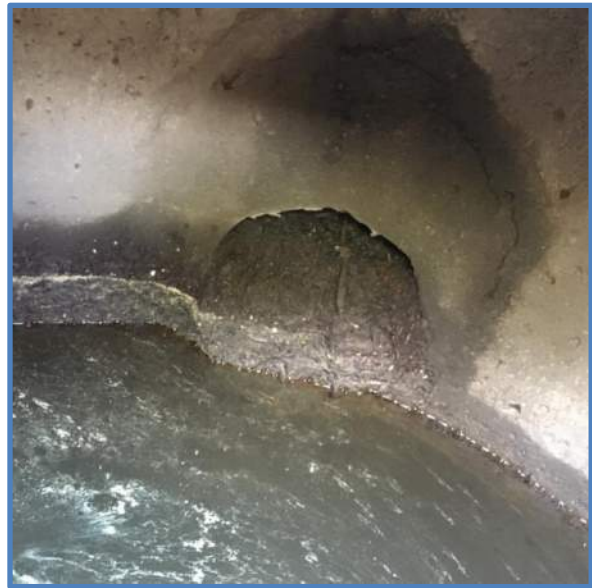
Photo 4 - Inlet Pipe & Pipe Penetration
