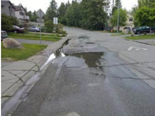
Ponding along the west side of Reflection Drive viewing north
