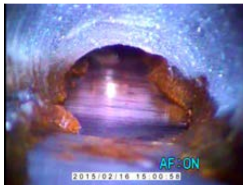
18-inch CMP storm drain in Reflection Drive (photo courtesy Steph Engineering, LLC)
