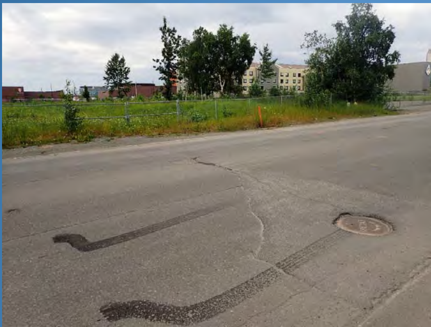
Lack of pedestrian facilities and pavement distress on E. 33 rd Ave
