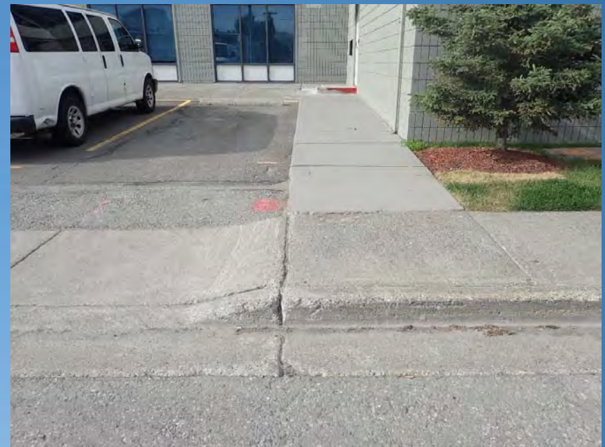
Non compliant driveway ramp on north side W. 32 nd Ave
